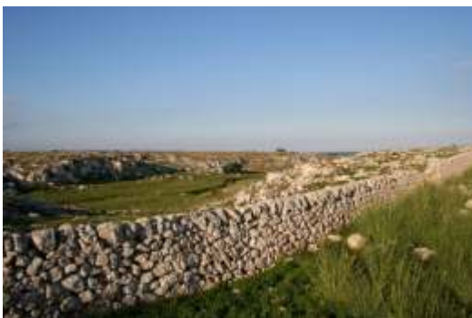
Contrada Cugni - boundary wall
