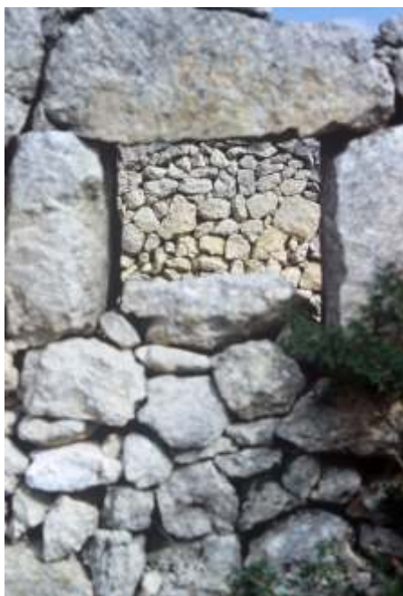
Drystone walls of a farm's ruin
